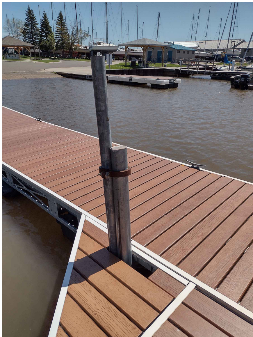
5 S2.0 EXISTING 45° CORNER W/ SLOTTED POCKET
