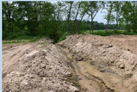
Stream restoration projects can reduce concentrated flow entering the channel by dispersing flow in the floodplain and increasing ground cover near the channel. Combining multiple concentrated flow points into a single concentrated flow point does not count as an improvement. The restoration activity must diffuse or capture the runoff. Example activities include filling ditches, removing pipes, routing concentrated flow into created oxbow ponds, and stormwater BMP's.
