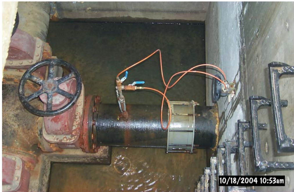
Figure 7-1. USFWS Siphon Well and Water Meter
