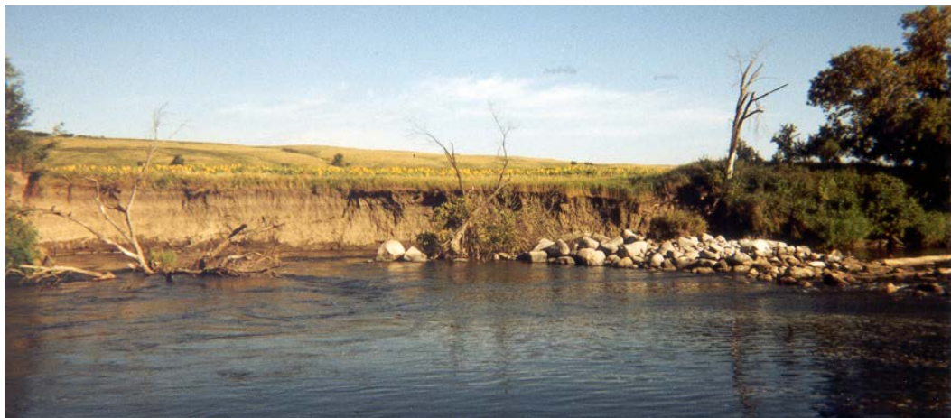
Figure 3-1. Scour of the Tailwater Gaging Location
