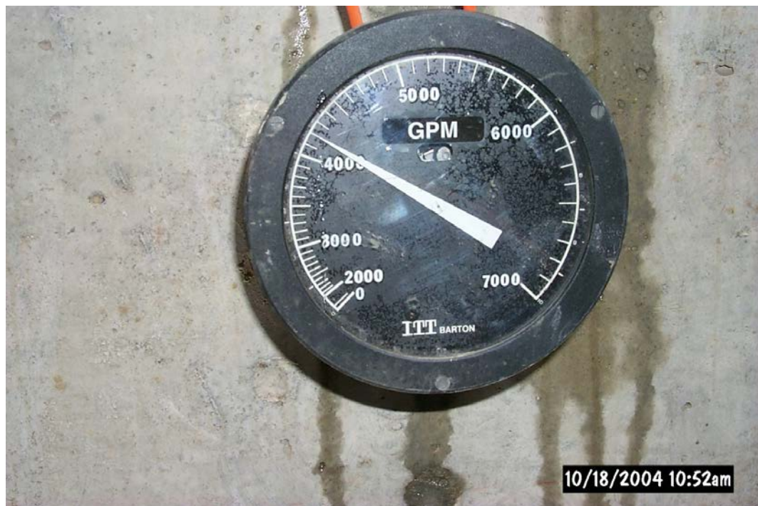
Figure 7-2. COE Water Meter to Monitor USFWS Demand
