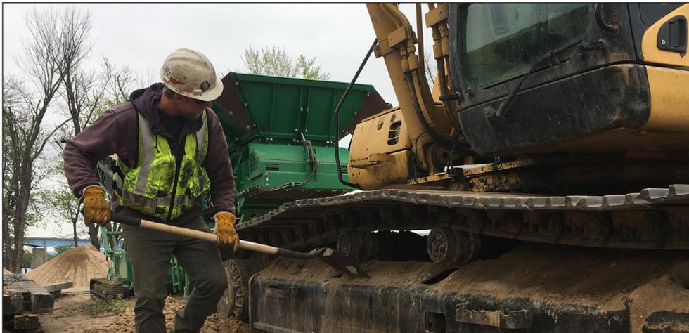
Scott Rolbiecki, operations, removes sand from the tracks of an excavator before dredged material placement at McGregor Lake. USACE photo by Nayelli Guerrero
