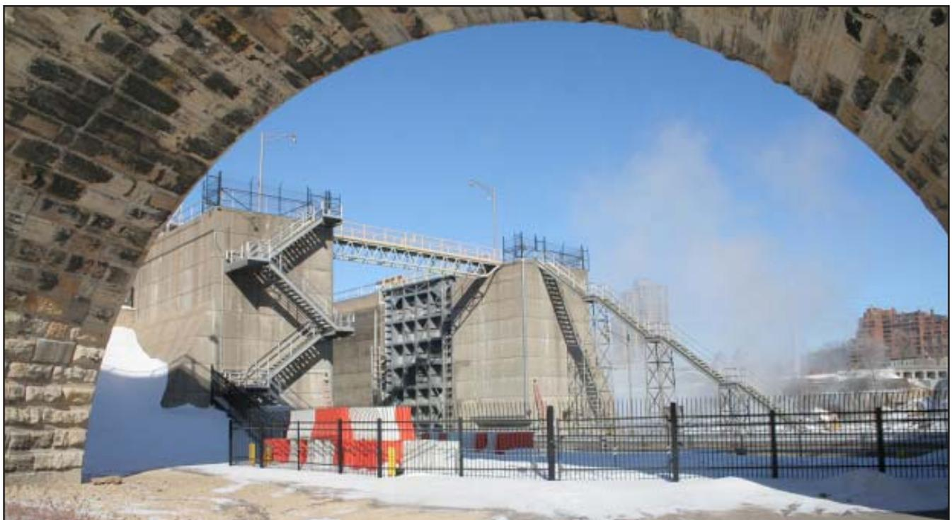
At right is the discharge point for Basset Creek tunnel. The Corps dropped the water level of the Lower Saint Anthony pool 13 feet to allow engineers to inspect the inside of the tunnel. The drawdown began Feb. 17 at 8 a.m. The Corps restored the project pool level Feb. 24 at 4 p.m.
