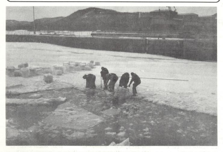
If you think you were cold this last winter, take a look at the work that was being done at Lock and Dam 6 in Trempealeau, Wisconsin. Lock personnel had to cut through ice 3 feet thick in the upper gate bay (110 feet by 60 feet) with chainsaws and ice chisels. The resulting 200 pound blocks were then dragged away with ice tongs to clear the way for opening the upper miter gates. Fortunately, they usually aren't frozen open as seen in this photo. Anyone interested in a job reassignment?
