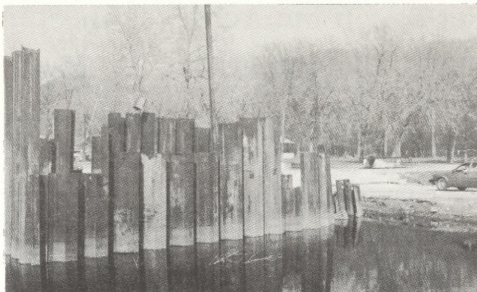
Steel sheet piling was used to dewater the backwaters of the Mississippi River.
