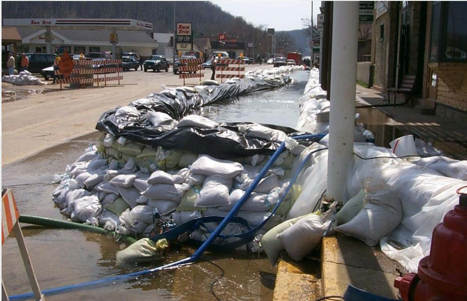
Sandbag ring levee with poly on inside face to prevent seepage
