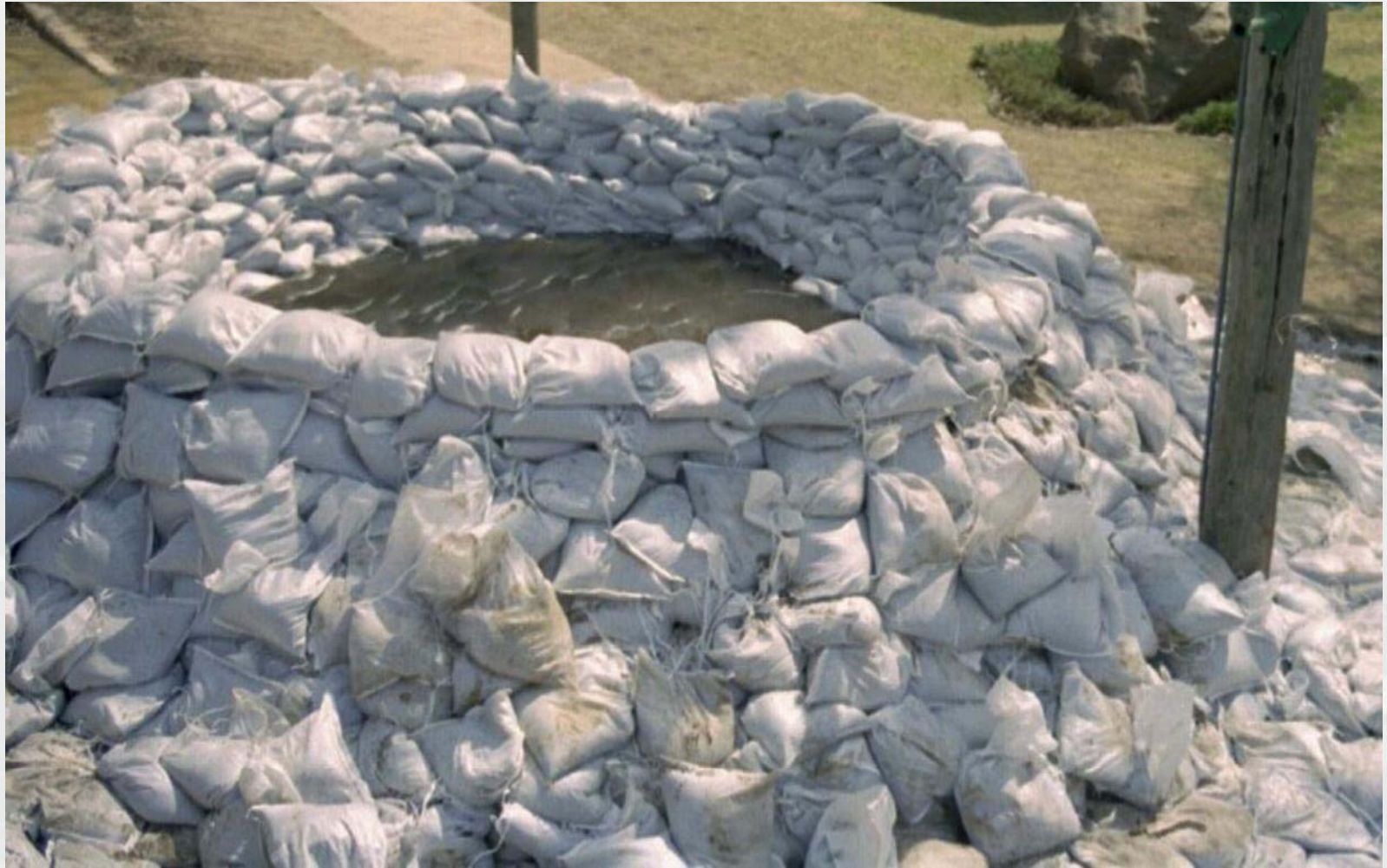
Sandbag ring levee to contain seepage
