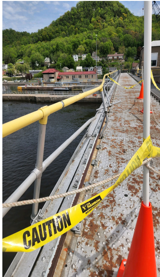
Dam service bridge (LD4)
