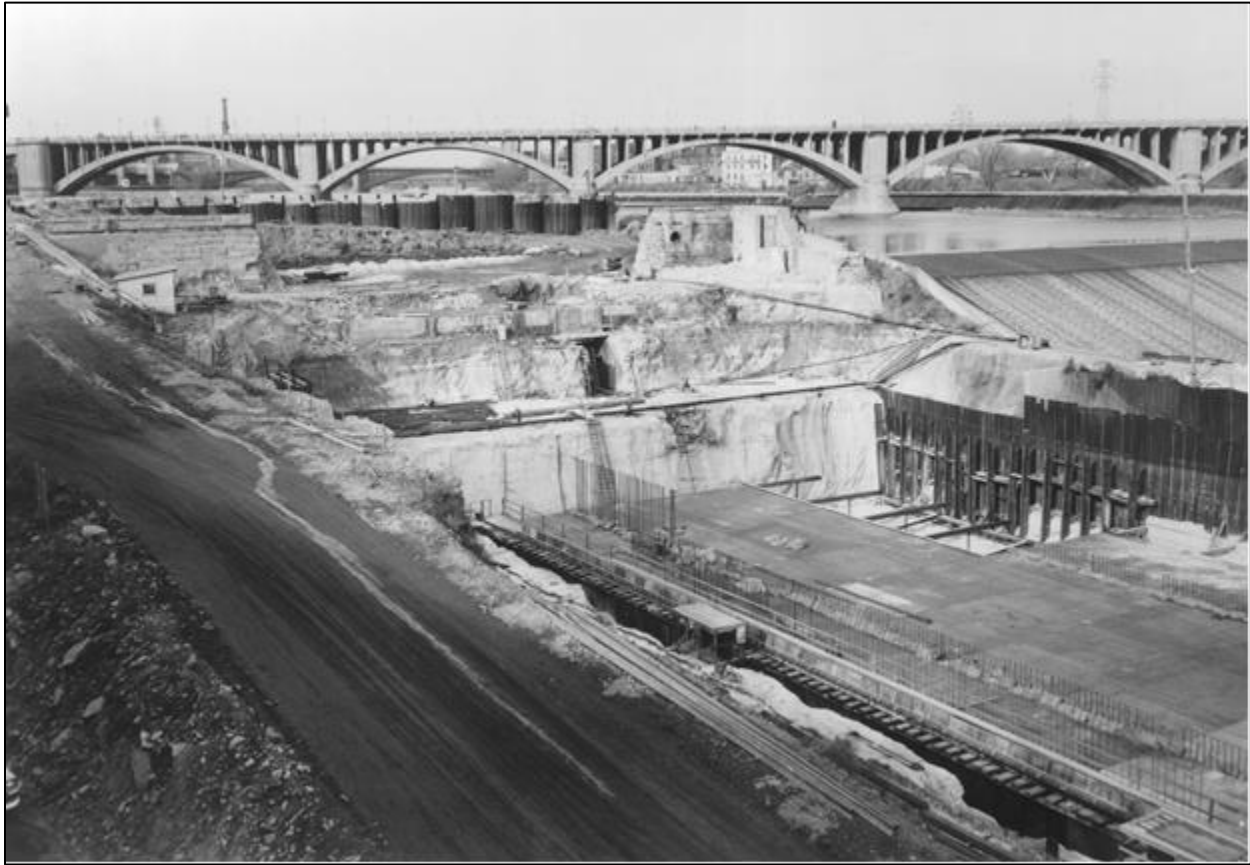
Figure 5-2. Upper St. Anthony Falls Lock Construction
