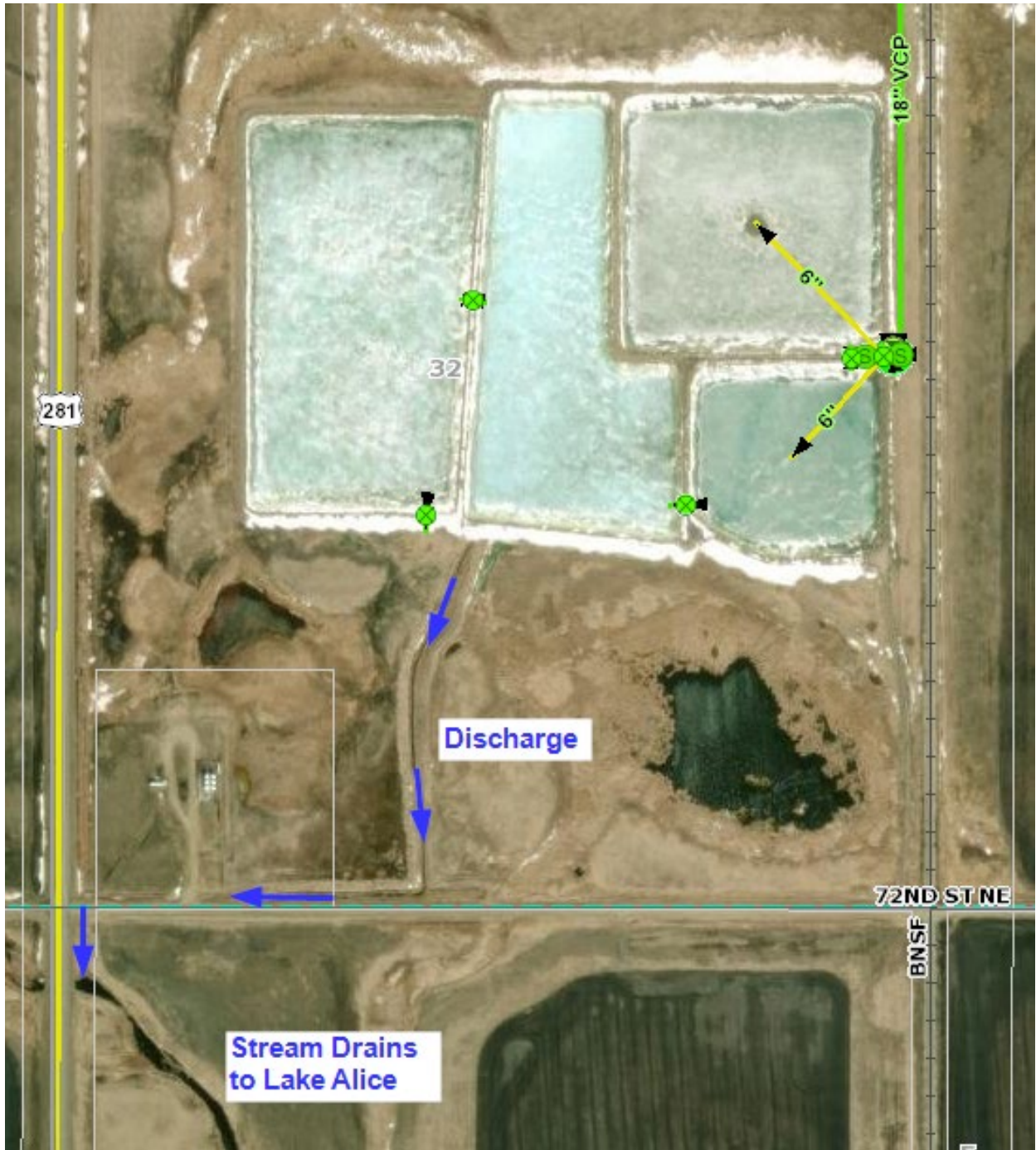
Figure 6. Wastewater Treatment Ponds
