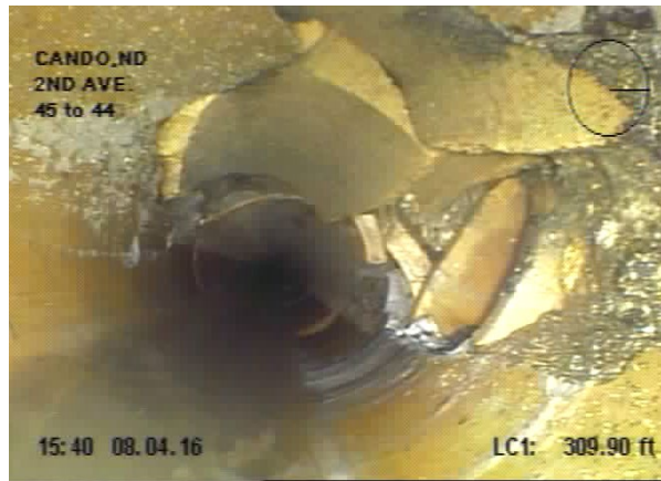
Top of Pipe is Broken and Missing
