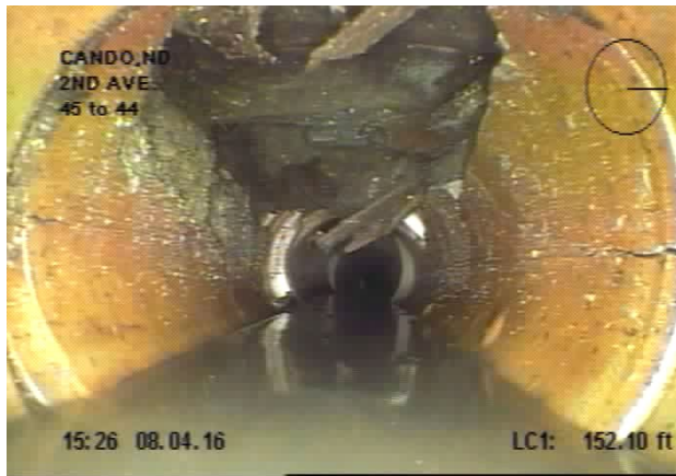
Top of Pipe is Broken and Missing
