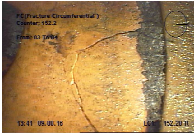
Fractures in Pipe Wall at Joint
