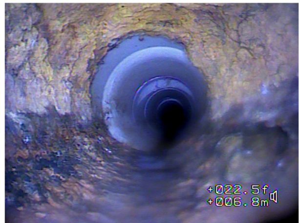
Figure 8: Transition from Cast Iron to New PVC – Unit 405E
