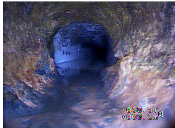
Figure 4: Transition from Cast Iron to PVC Piping – Unit 412W
