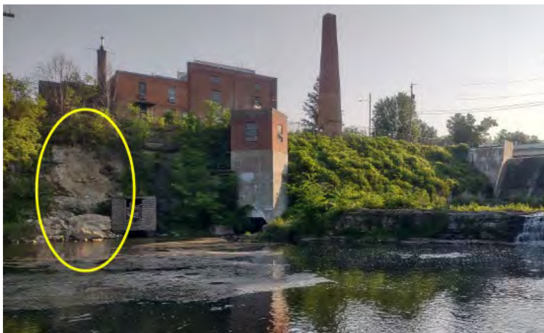
Figure D-7: Photo looking north to the alluvial valley rock wall downstream of the Junction Falls Dam showing the scar from a rock slide, inside of yellow oval.
