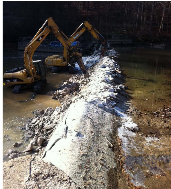
Figure 23. Jackhammers comb through a rebar reinforced concrete spillway during dam demolition (photo Inter-Fluve).
