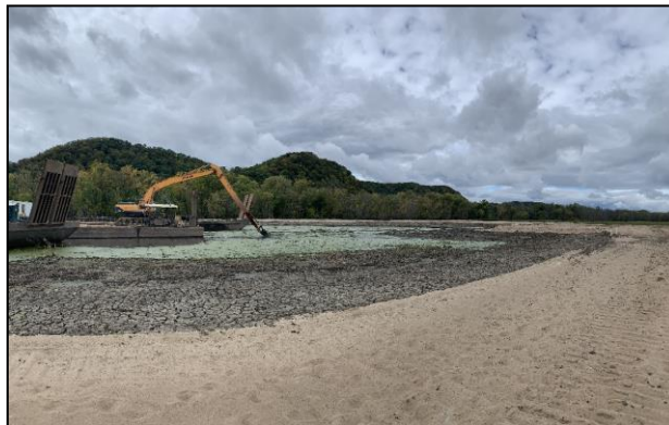
Photo 6. Example of mechanical dredging.
