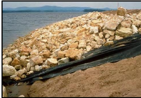
Photo 3. Example of shoreline stabilization using riprap.
