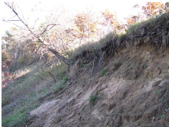
Erosion of the bank along the Red Cedar River adjacent to Dunn County Road M.
