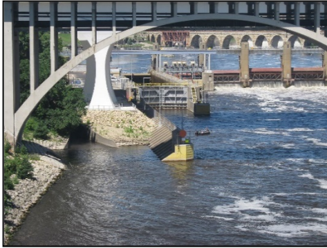
Lower St. Anthony Falls Lock and Dam.
