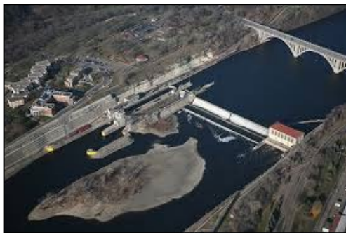
Lock and Dam 1.
