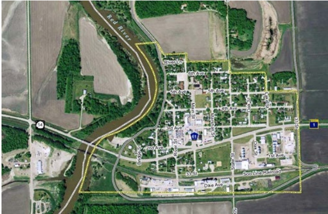
Construction of Corps approved major levee modifications to the Oslo, Minnesota, levee project was completed in 2013.
