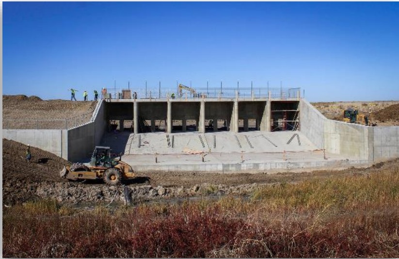
Marsh Lake water control structure
