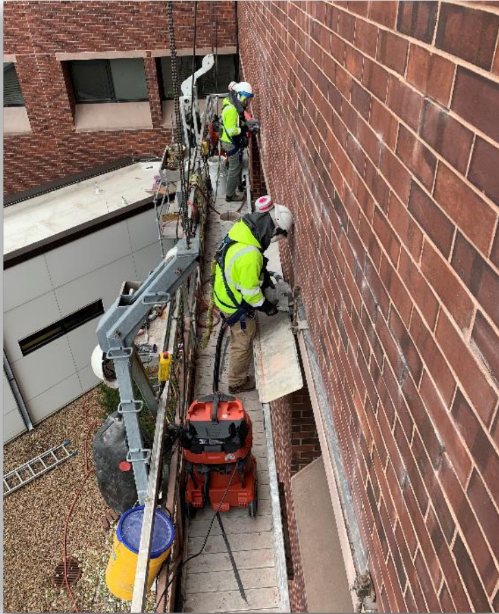
Repairs at the Minnesota Veterans Affairs hospital
