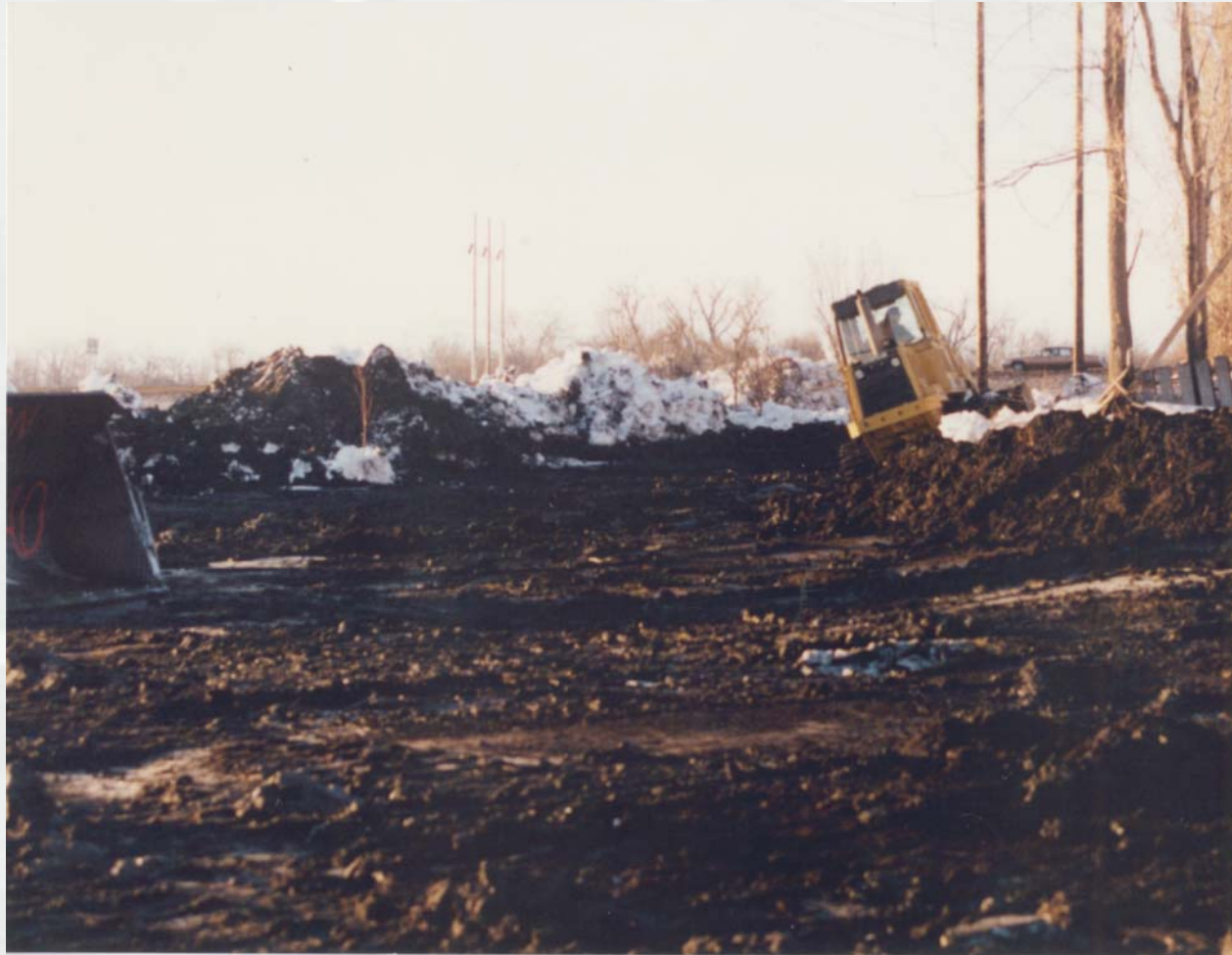
Stripping topsoil prior to placing levee fill
