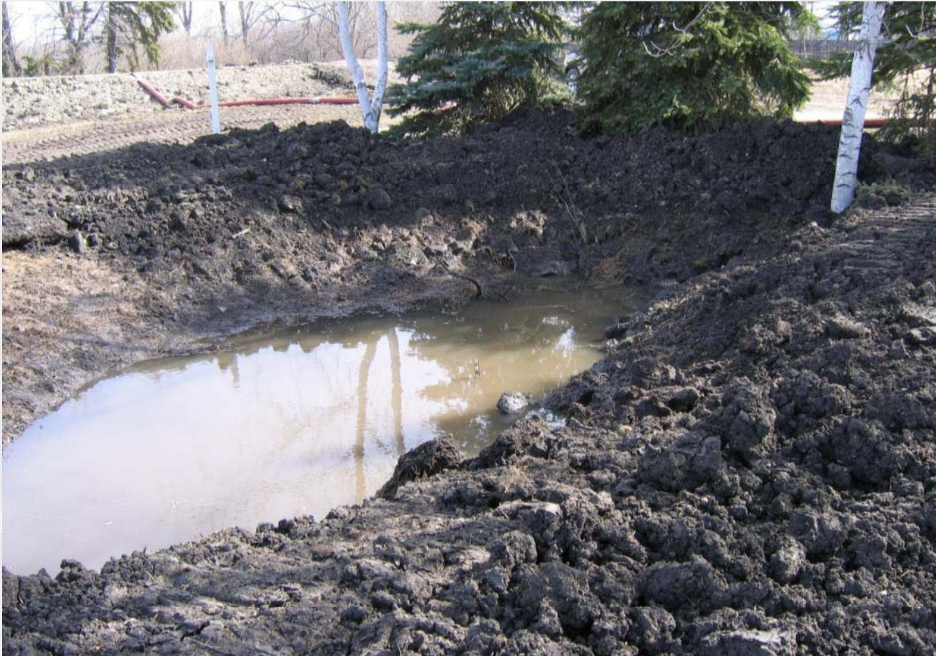
Ring levee constructed to contain seepage on the landside of levee
