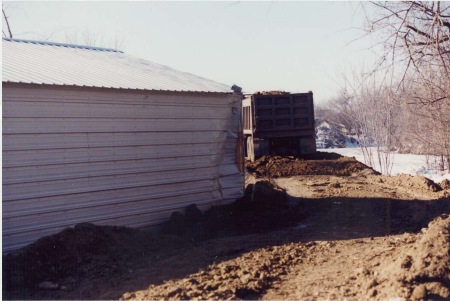
Garage damaged during levee construction
