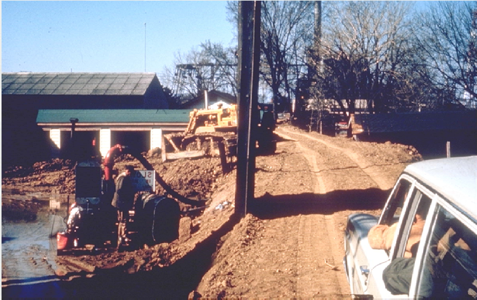
Pumping interior runoff from landside of levee
