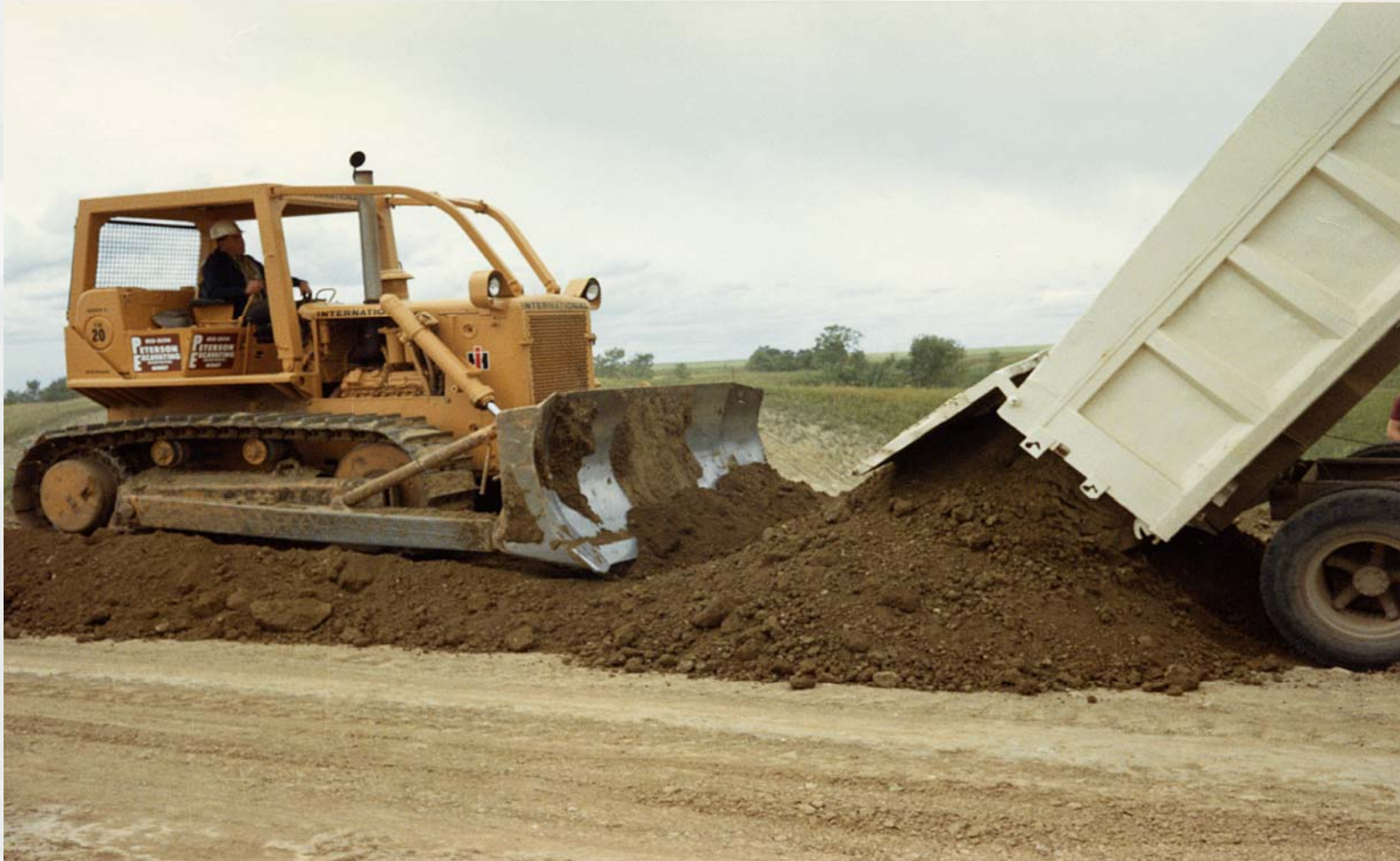
Spreading and compacting clay fill for levee
