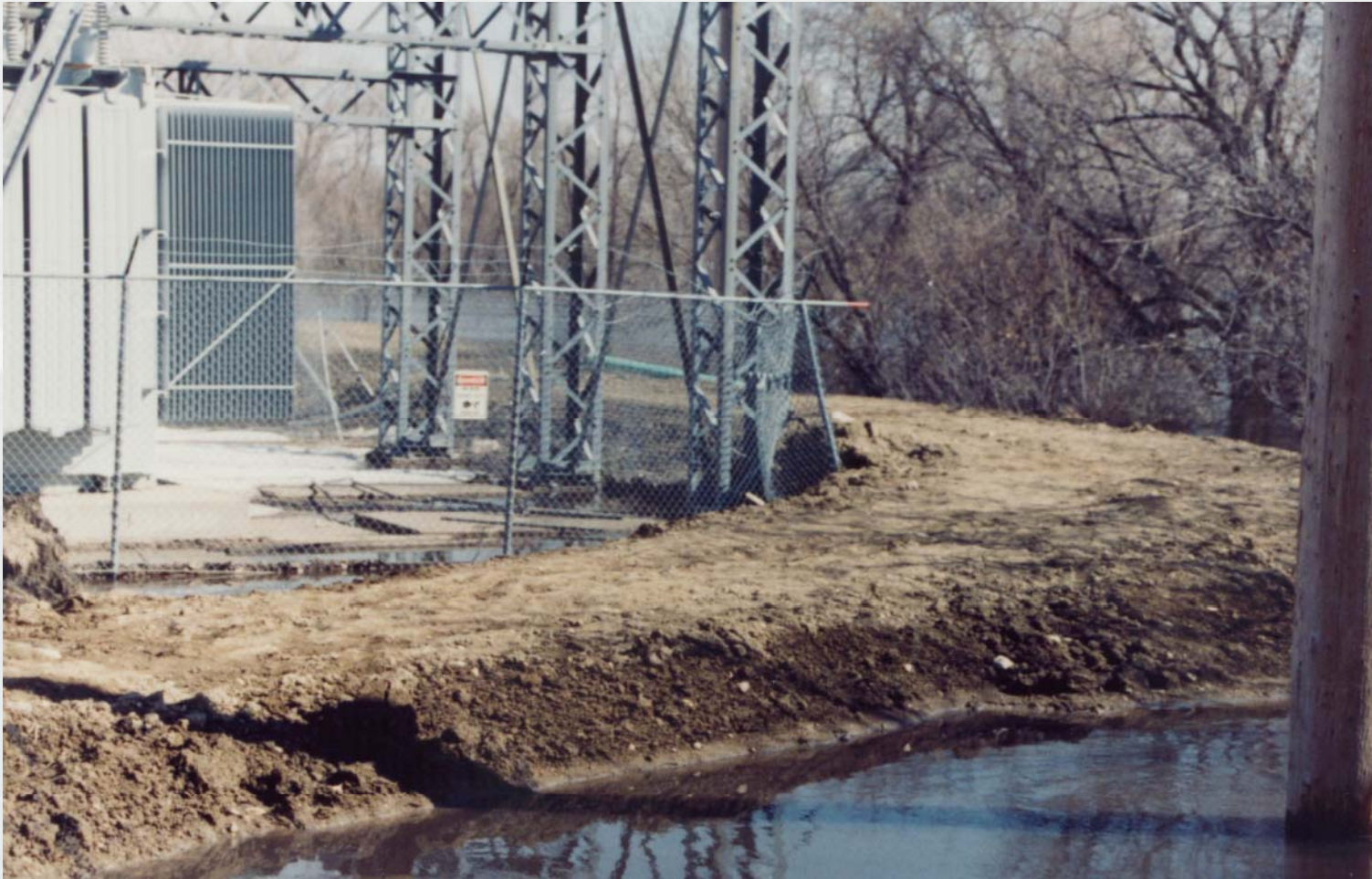
Levee constructed adjacent to electrical substation
