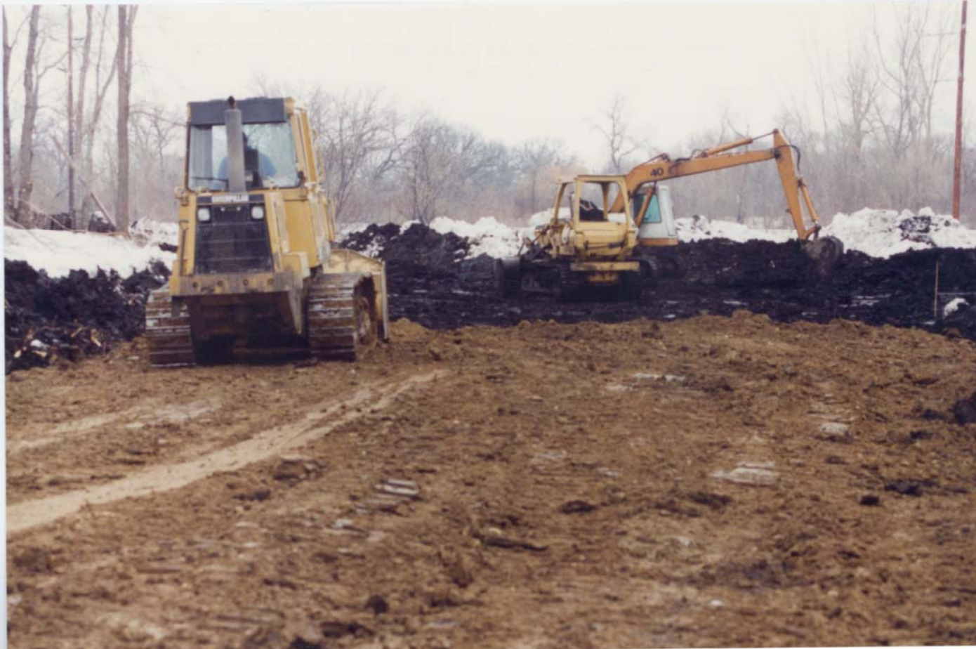
Placement of clay fill over stripped levee foundation
