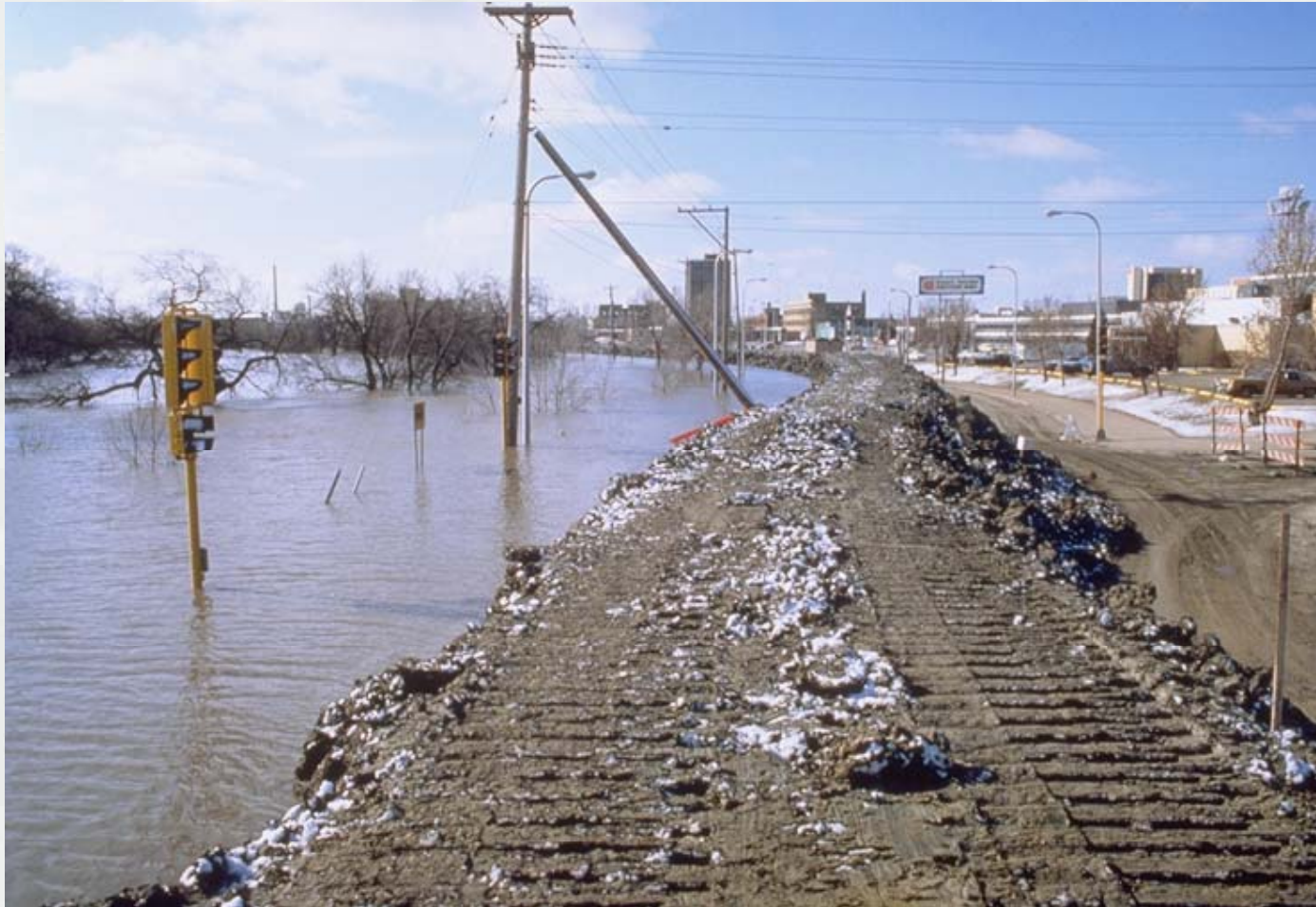
Finished emergency clay fill levee
