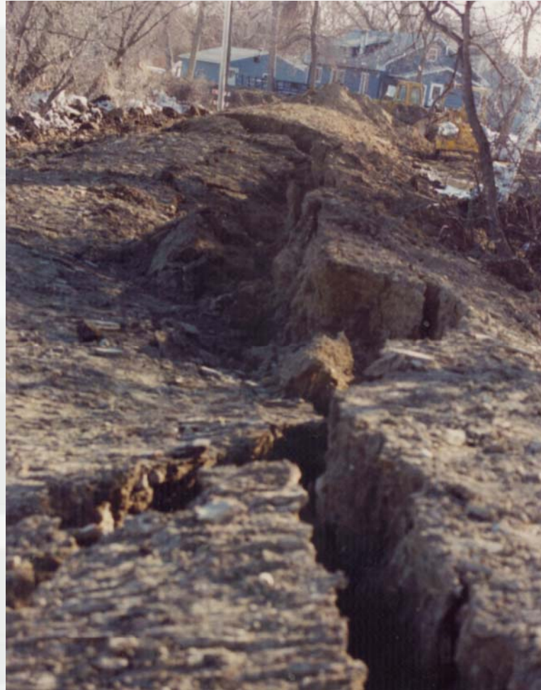
Levee stability failure
