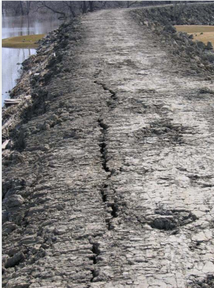
Cracks developed on levee slope
