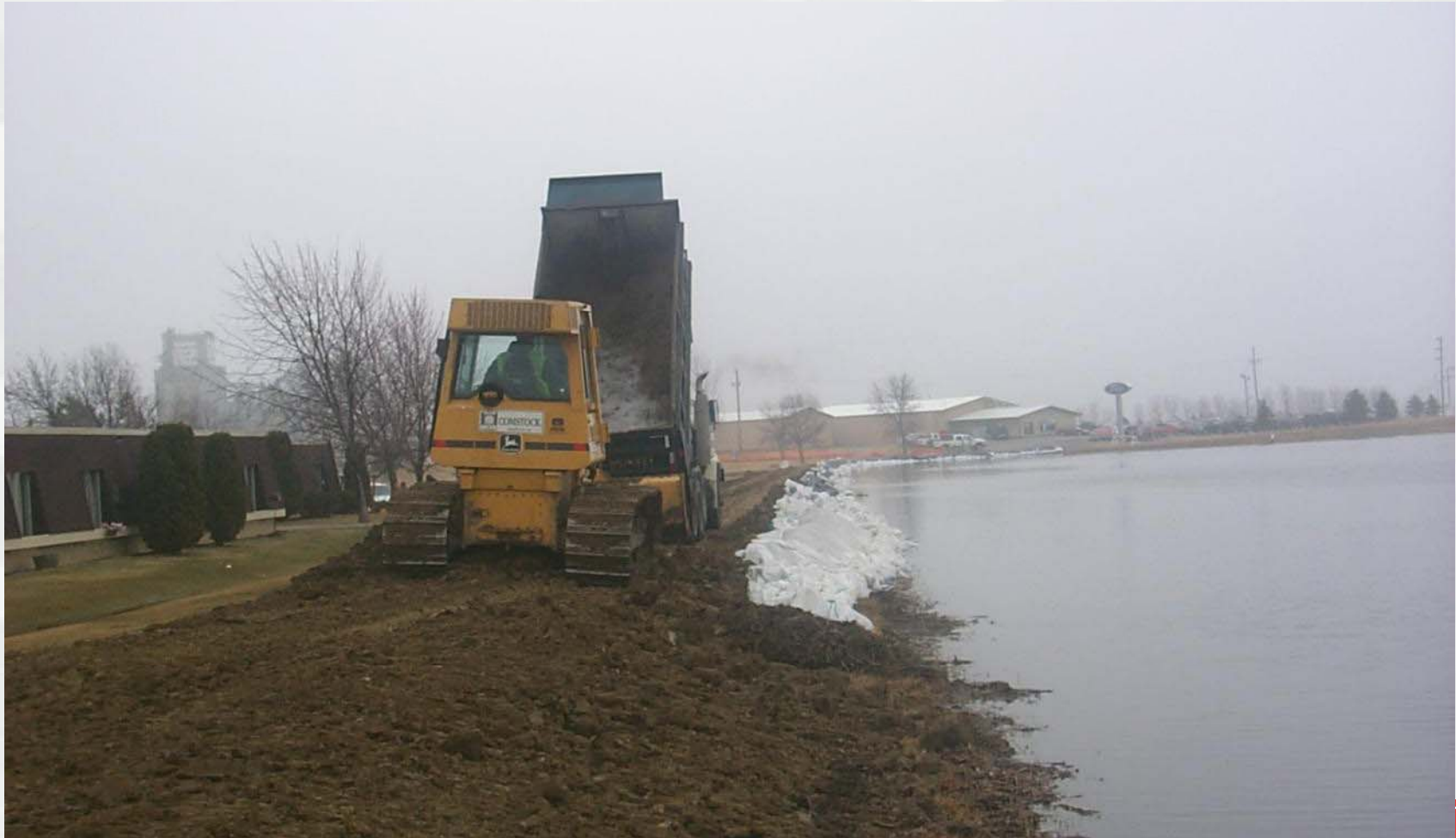
Placement and compaction of clay fill
