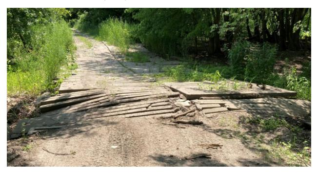
Figure 17 Texas crossing (damage, including erosion, concrete loss, debris impaction)
