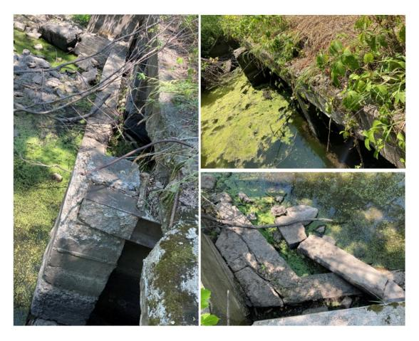
Figure 18 Culvert (damage, including exposed reinforcing steel and significant section loss)
