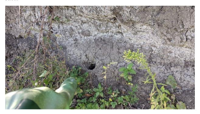
Figure 28 Animal burrows present in current slope along Reach 2
